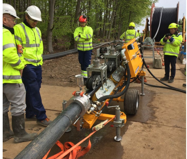
Fig. 6: Installation of the cable in Copenhagen
