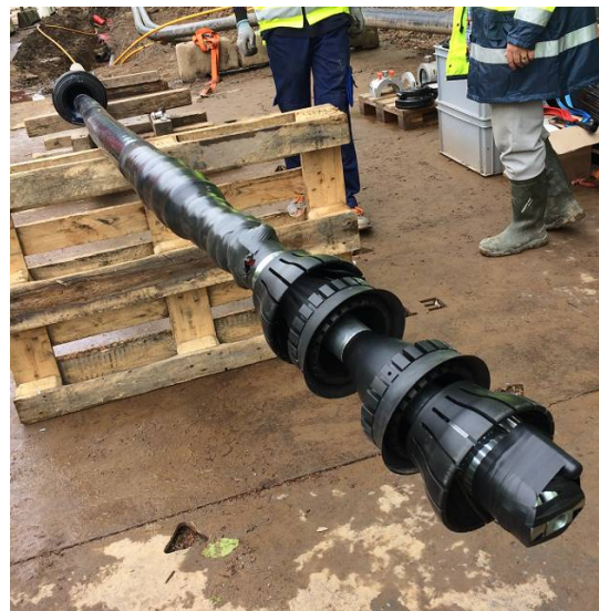
Fig. 3: Rear end of cable prepared for FreeFloating
