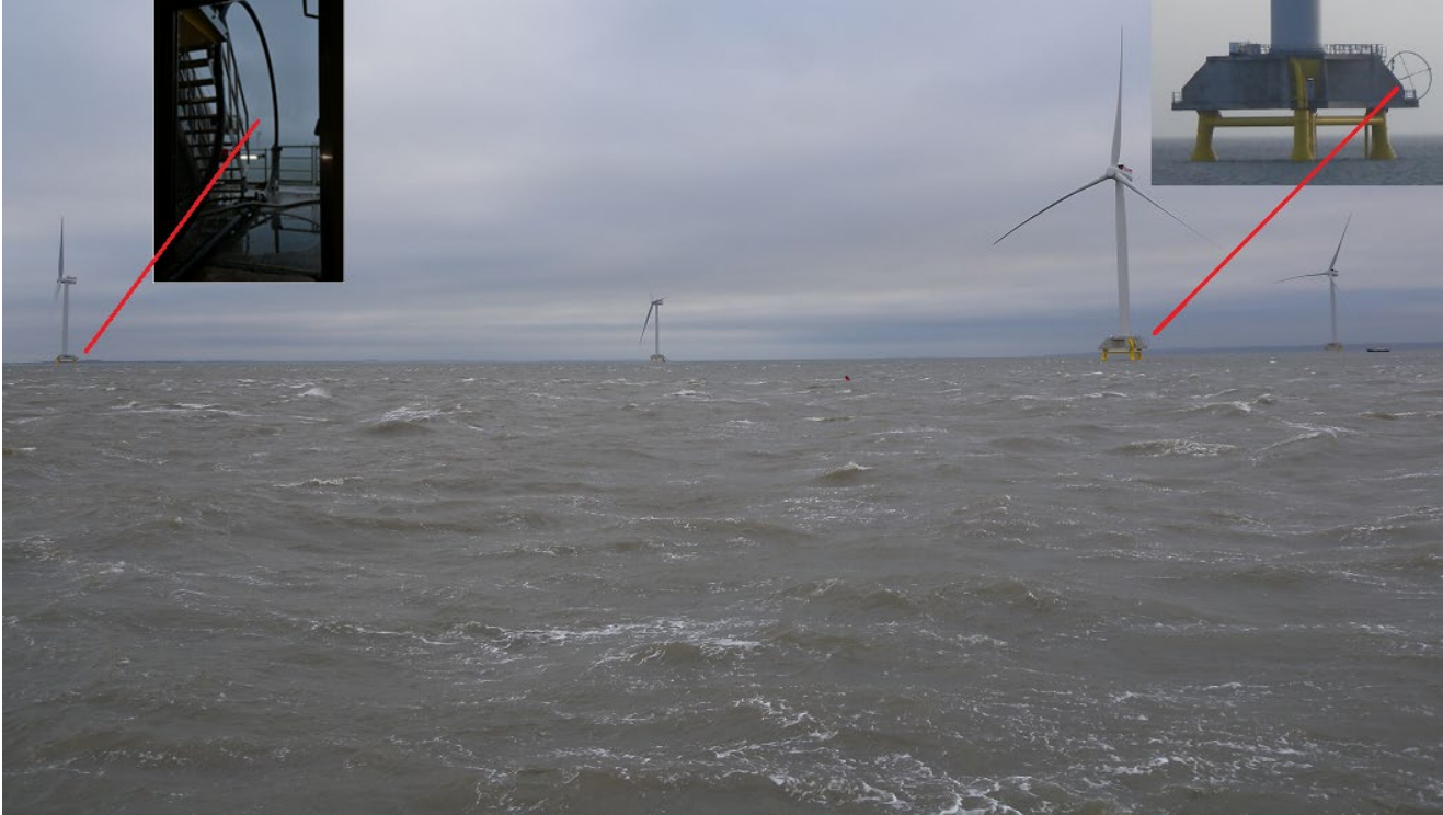
Fig. 7: Nissum Bredning Offshore Wind Farm, with details of FreeFloating return loops
