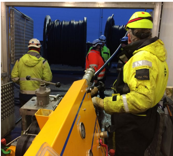
Fig. 8: Installation of the cable at Nissum Bredning
