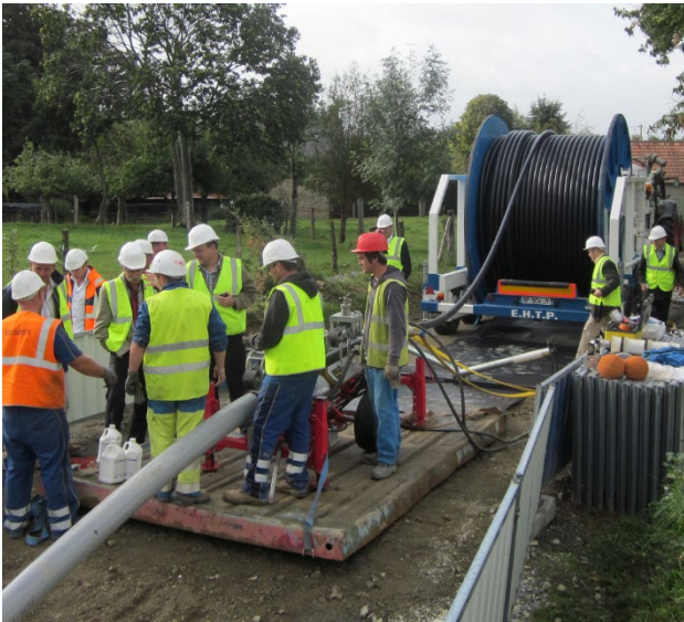
Fig. 2: Cable installed by using water
